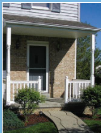
ROOF SUPPORT COLUMNS
