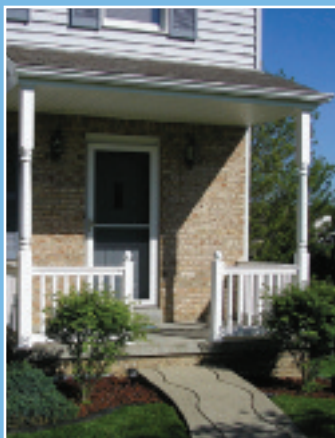
ROOF SUPPORT COLUMNS
